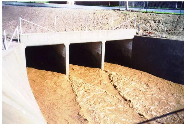
*Figure 1: Supercritical flow with hydraulic jumps under a bridge*
